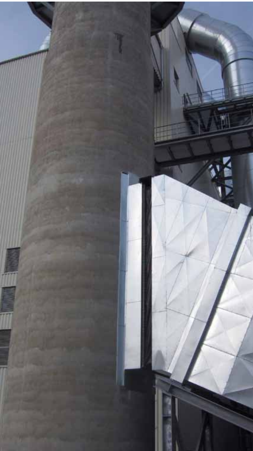
KOREMA® expansion joint fitted between induced draught fan and stack
